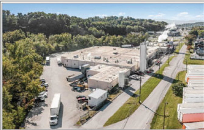
225 Commonwealth Avenue Extension – Bristol, VA
